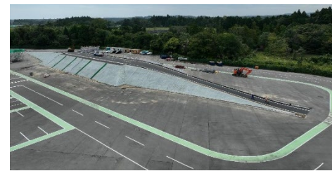
Demonstration test of road fill in the Interim Storage Facility (Okuma Town)
