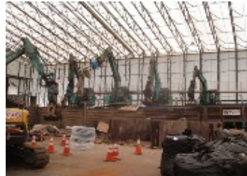
Soil reception / separation facility of Interim Storage Facility (Okuma Town)
