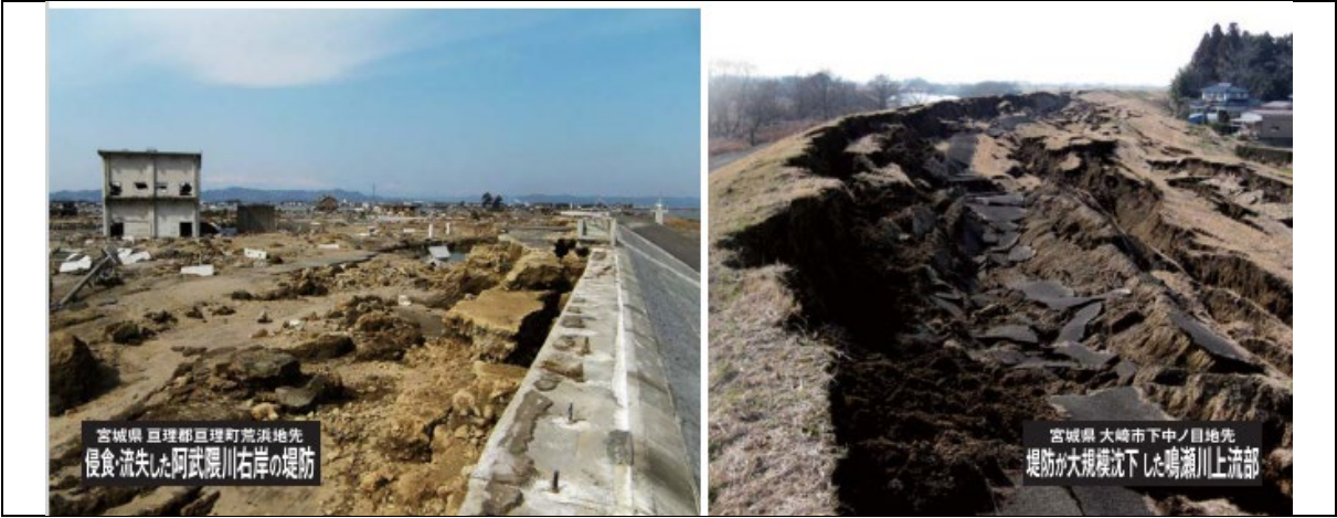
Figure 5-6-4 Examples of damaged river levees
