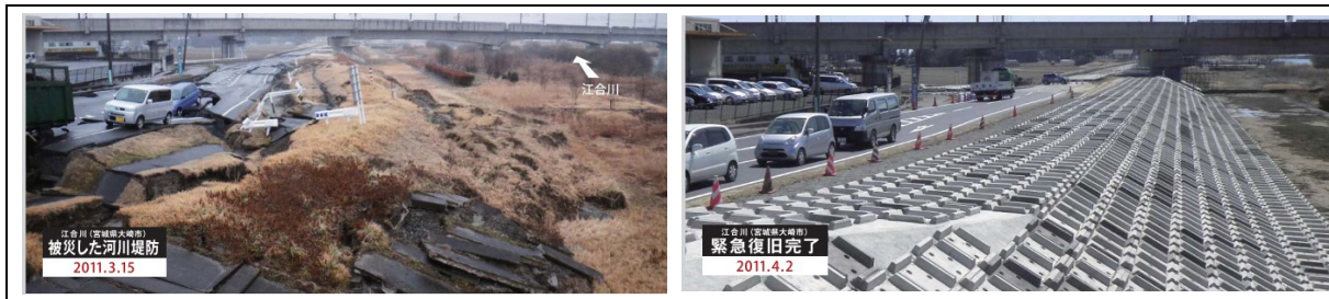
Figure 5-6-7 Example of emergency restoration work for river levees (Eai River in Osaki City, Miyagi Prefecture)
