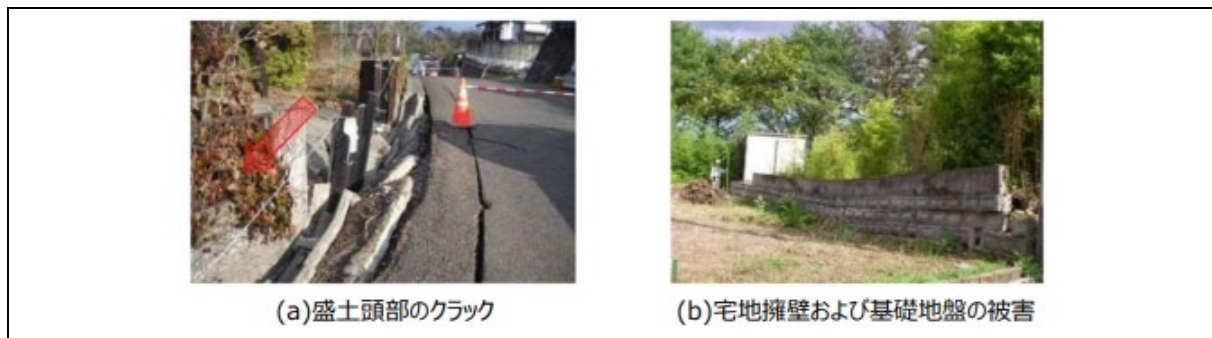
Figure 5-4-2 Photographs of Areas Where Entire Embankments Sustained Deformation Damage
