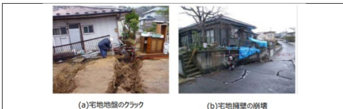
Figure 5-4-6 Photographs of Areas Where Combined Deformation of Entire Embankments and Terraced Areas Occurred
