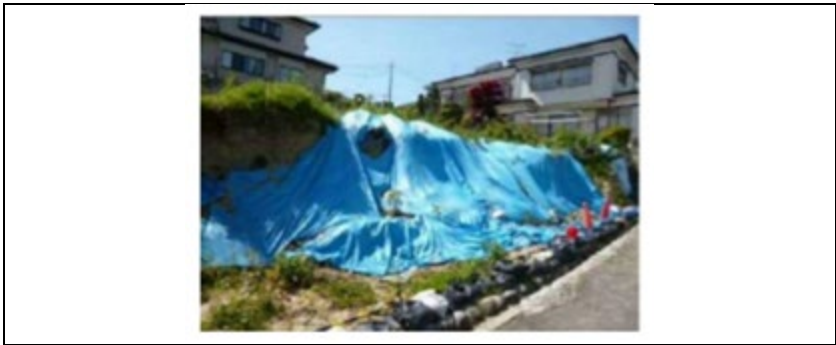
Figure 5-4-4 Photograph of an Area Where Terraced Areas Sustained Deformation Damage
