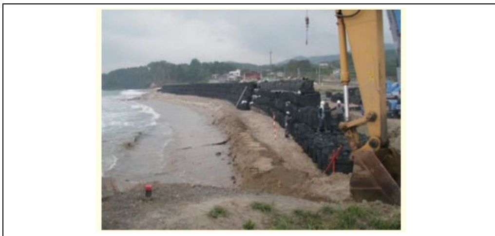
Figure 5-12-2 Emergency construction using large sandbags
