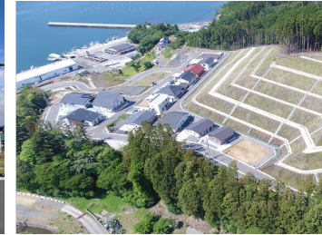
Relocation to higher ground in Ishinomaki City, Miyagi Prefecture (Oginohama area)
