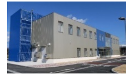
Collaborative Laboratories for Advanced Decommissioning Science
