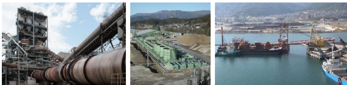
Photos: Kiln No.5 undamaged by the tsunami (left), installation of salt removal equipment (center), wide-area receipt of waste by ship (right) (Source: Taiheiyo Cement Corporation's Ofunato Plant)
