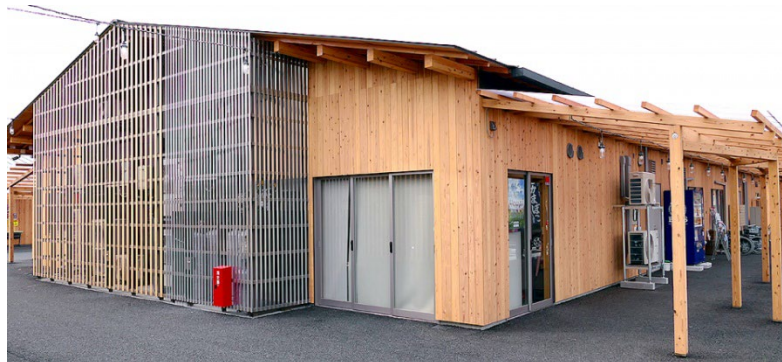
Photo: Shopping street facilities designed using Bijin-sugi (Source: Minamisanriku Sun Sun Shopping Village website)
