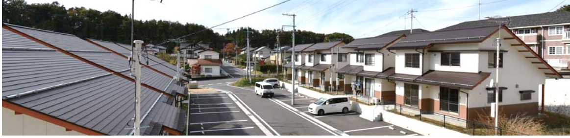
Photo 2: Exterior view of Ishizaki Housing Complex
