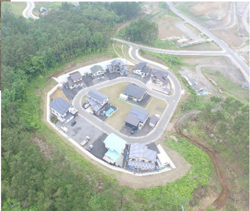
Maita district (project on promoting group relocation for disaster prevention)
